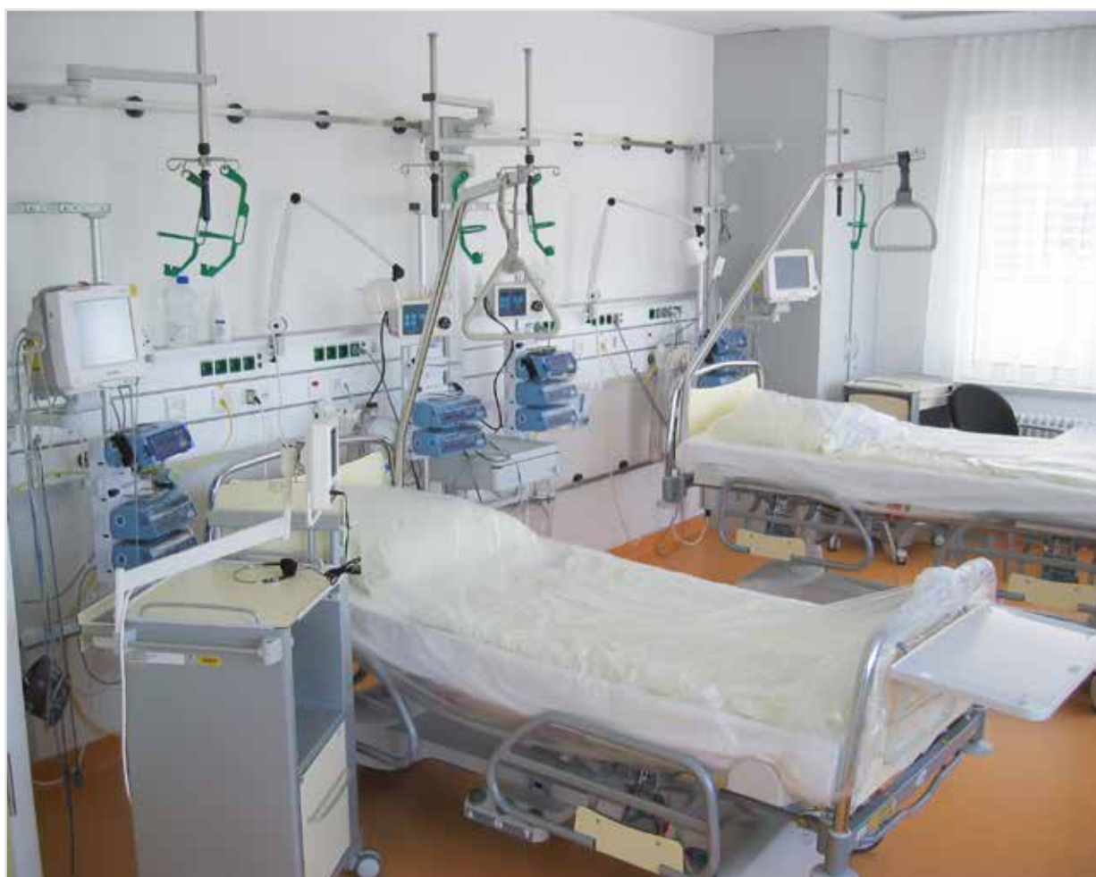
Fixing to wall supply duct and standard runner on the intensive-care station
